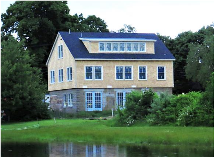
The exterior was fully shingled in early June.
