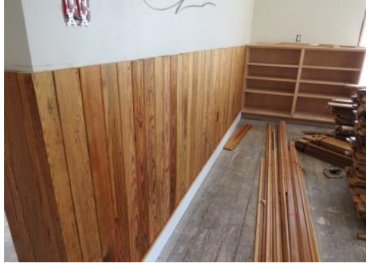
Charley Appleton delivered the finished wainscoting boards, reclaimed from the old attic. Workers began installing the elevator mechanisms and plumbers installed the sinks and composting toilets.
