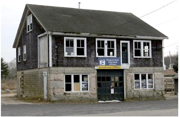
The Head Garage before renovation.
